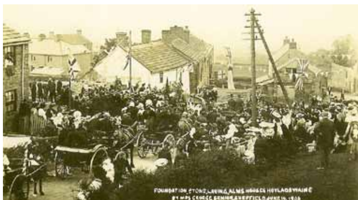
Laying the foundation stone for the almshouses by Mrs Senior (16 June 1906) Courtesy of Hoylandswaine History Group
