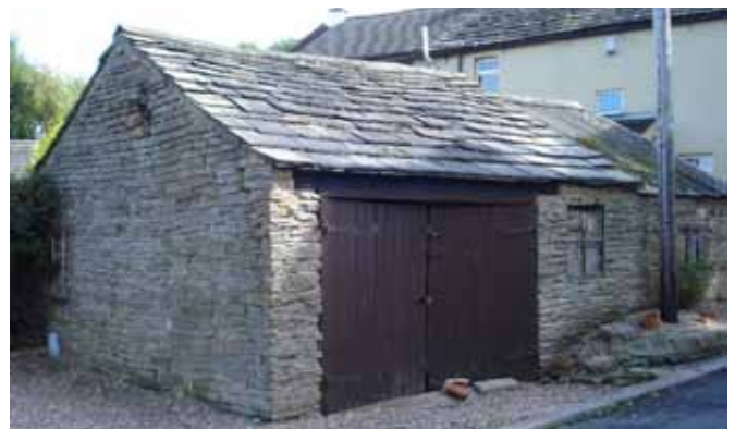
Former nail forge on Cooper Lane, now a garage © Jenny Lunn
